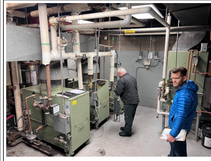
Boilers manufactured in 1970. Three used. Could replace with two. Two hot water makers use hot water from the boilers. One gas fired hot water gives quick delivery but might be replaced.
