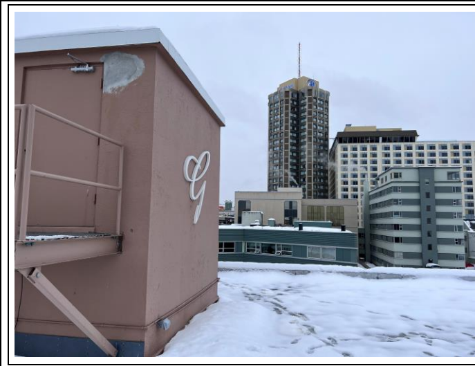
Elevator room above shaft. Membrane roof covering with turbine vents
