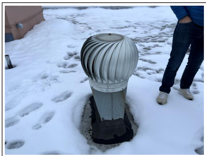
Elevator room above shaft. Membrane roof covering with turbine vents
