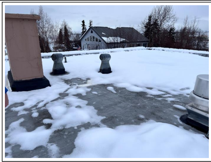
Elevator room above shaft. Membrane roof covering with turbine vents
