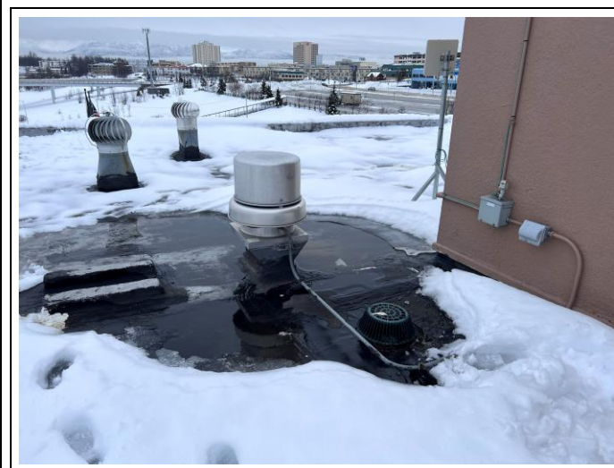
Elevator room above shaft. Membrane roof covering with turbine vents
