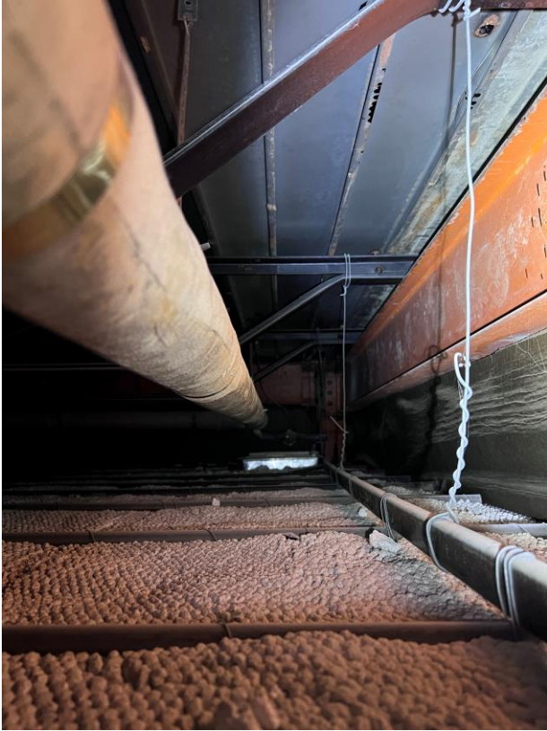
2' space above ceiling to underside of roof deck
