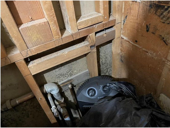
Replace the inexpensive Oatey brand air admittance valve with a Studor type
