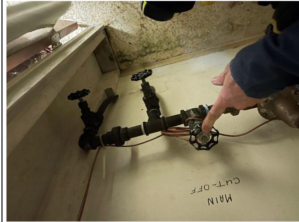
Finger points to your inside main shut off valve. Leave the others for circulation.
