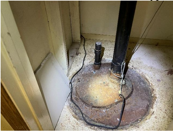
Replace the inexpensive Oatey brand air admittance valve with a Studor type
