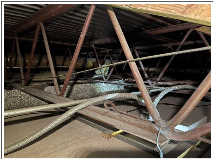
Mechanical and structural items in the way of a elevator installation on the south side hall.
