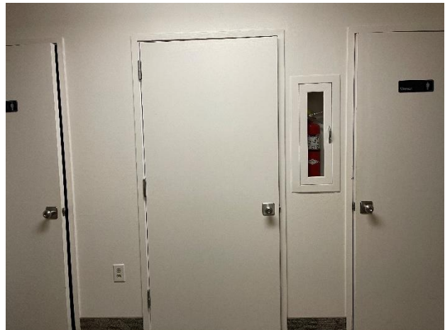
East side of south entry viewint restroom and janitor closet.
