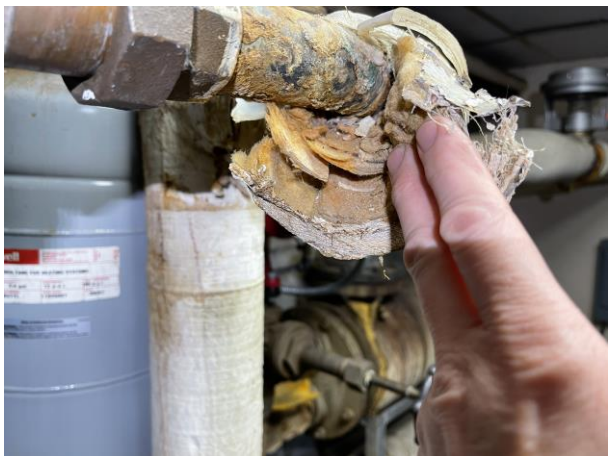
Insulation on pipes appears to be only fiberglass not asbestos.
