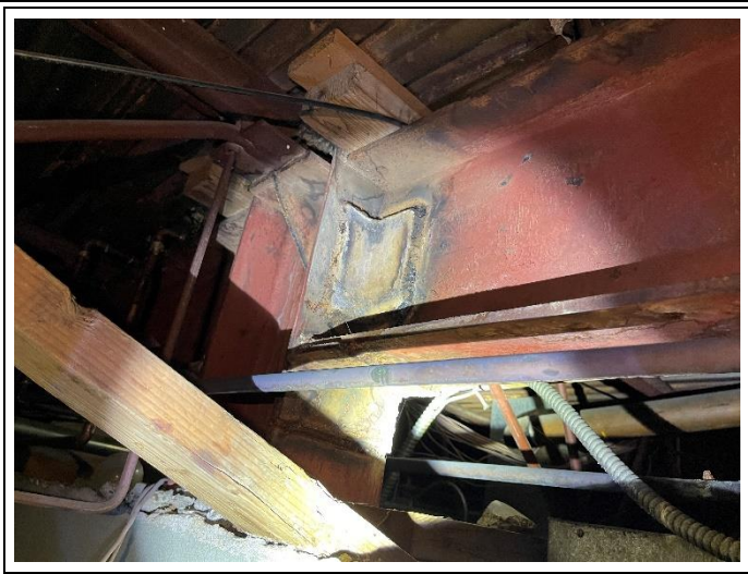
Mechanical and structural items in the way of a elevator installation on the south side hall.
