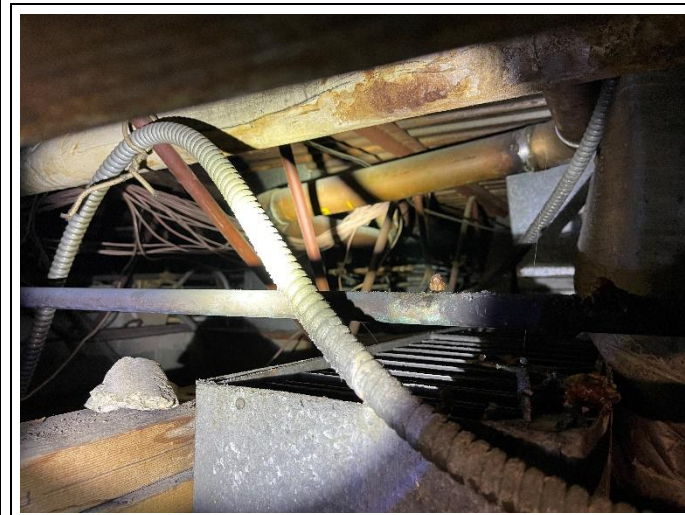
Mechanical and structural items in the way of a elevator installation on the south side hall.
