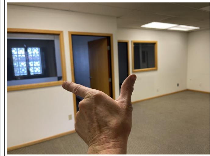
Windows within 24" of doors are to be safety glazing. Potable water temperature good just below 120F
