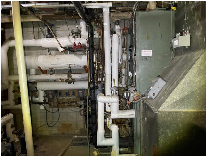
Insulation on pipes appears to be only fiberglass not asbestos.
